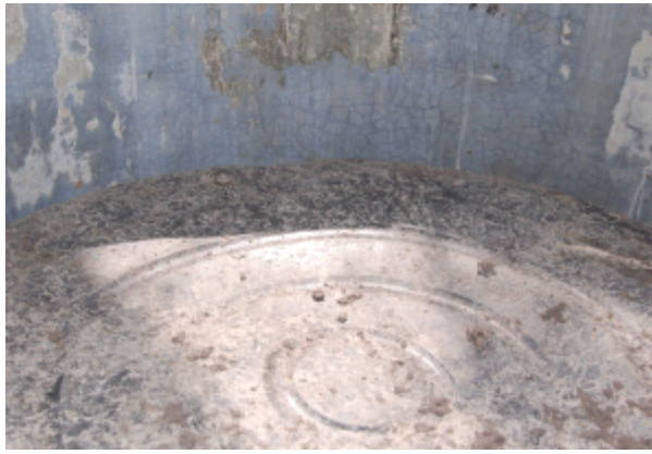
Fig III Gas dome in water jacket
