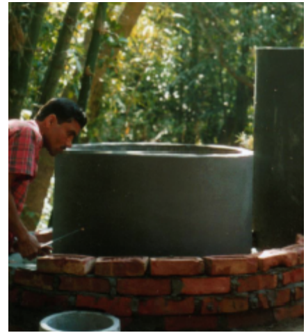
fig IV Construction of a water jacket plant (In the foreground the large inlet).
